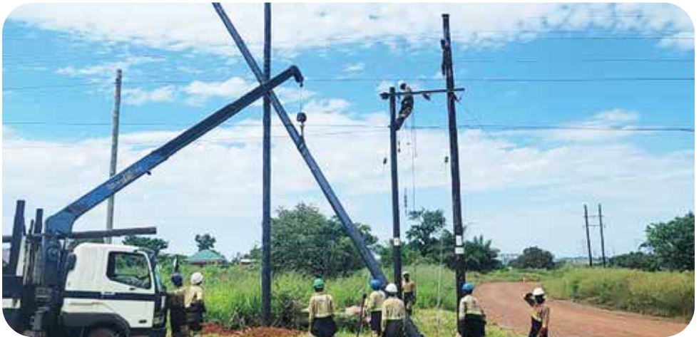
Expert powerline construction – bringing electricity to urban and rural areas.
